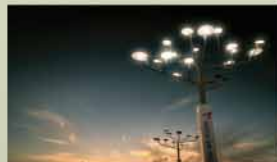
Installation of Solar energy streetlights in Angkor Wat
